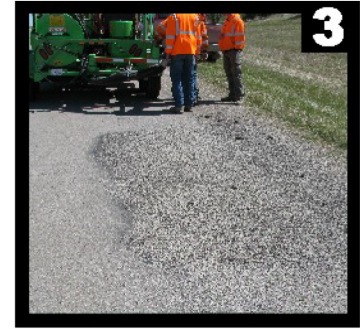
Cover With Dry Aggregate
