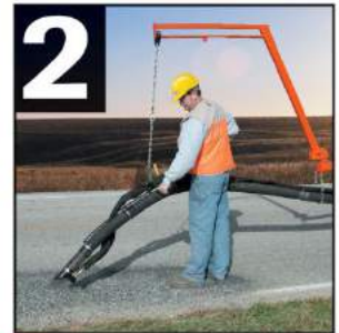
2 Apply tack coat to area to be repaired.
