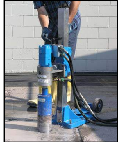
CD616 HydraCore Drill cutting a concrete slab
