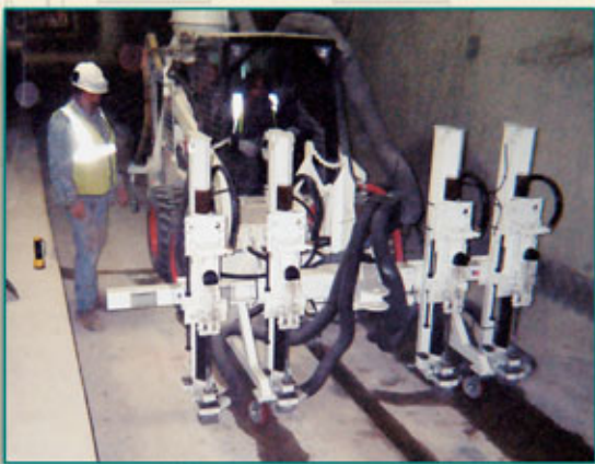
A-4 Vertical Equipment mounted drill used in tunnel construction.
