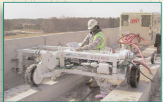
A-4S Core Drill used for light rail construction.
