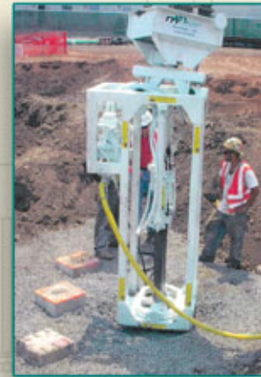
A-2 Vertical Equipment mounted drill used for drilling on foundations.
